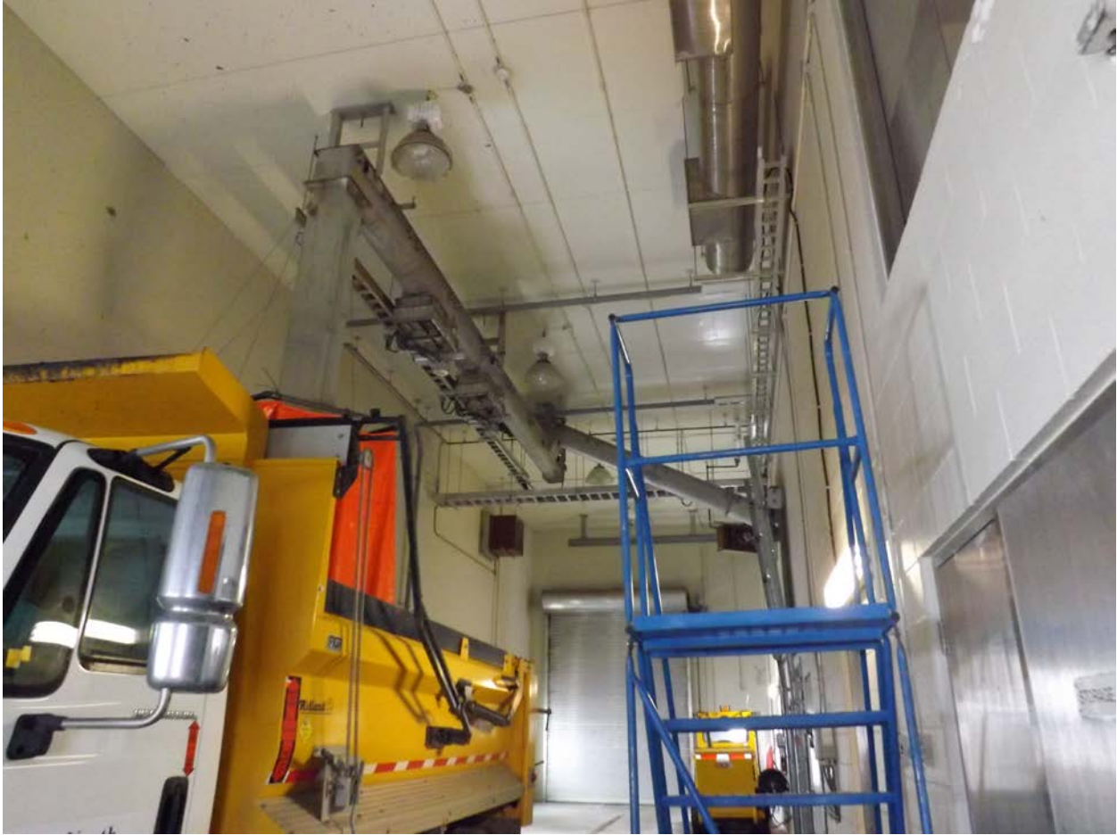
Figure 1: Sludge building before being retrofitted with Lystek system
